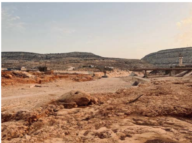
Figure 3. One of the Derna's bridges destroyed.
